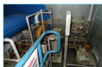
Lube Oil Skid with De humidifier Filter Housing
